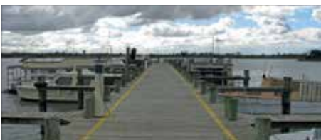
Berthing at a jetty
